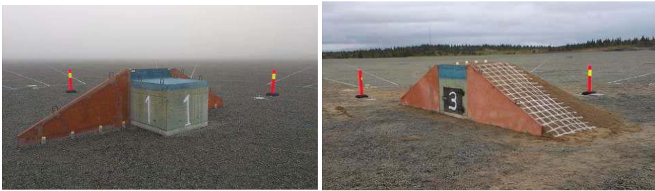
Figure 5 Construction of the 1/5 th scale test structure.
