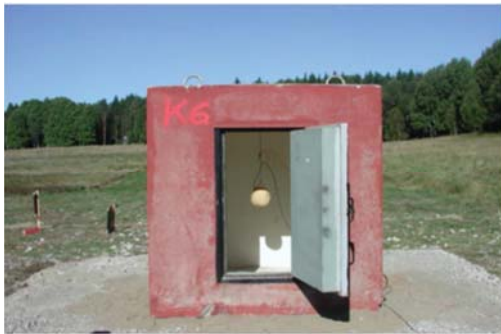
Figure 14 The Kasun structure with its heavy door.
